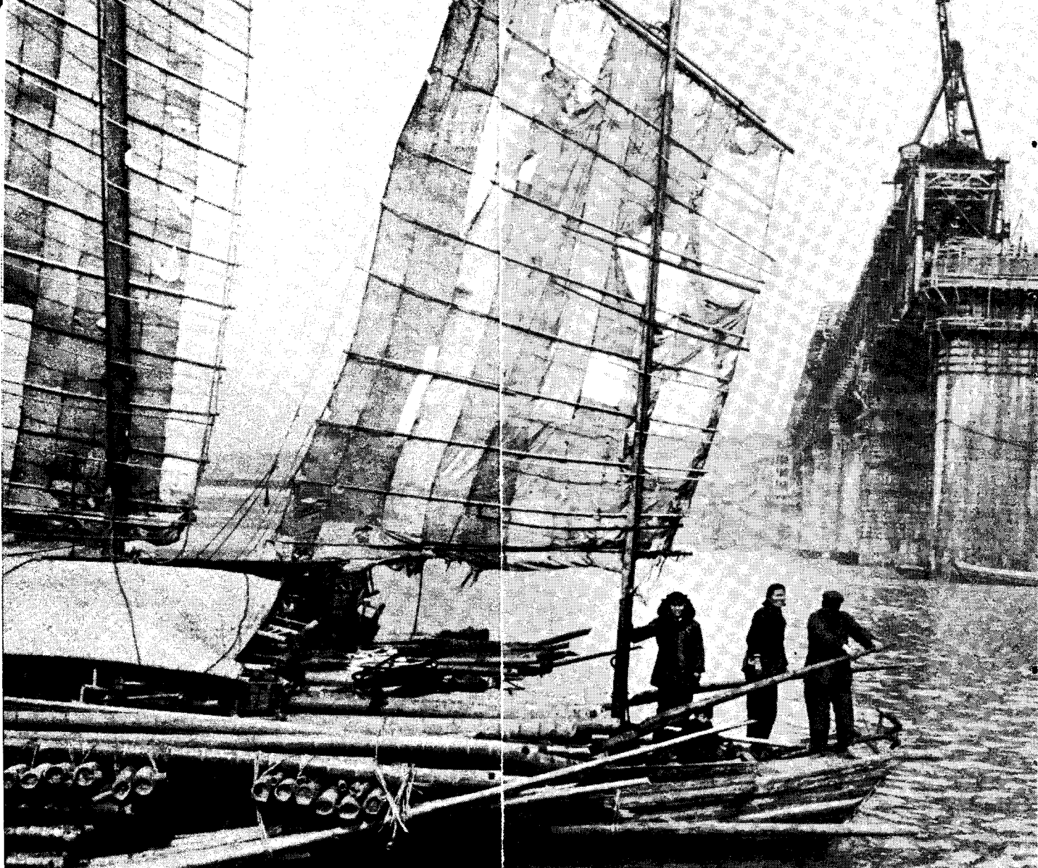
Building a bridge over the Yangtze (Yellow) River. Mao referred to the Yangtze as the spine of China.
