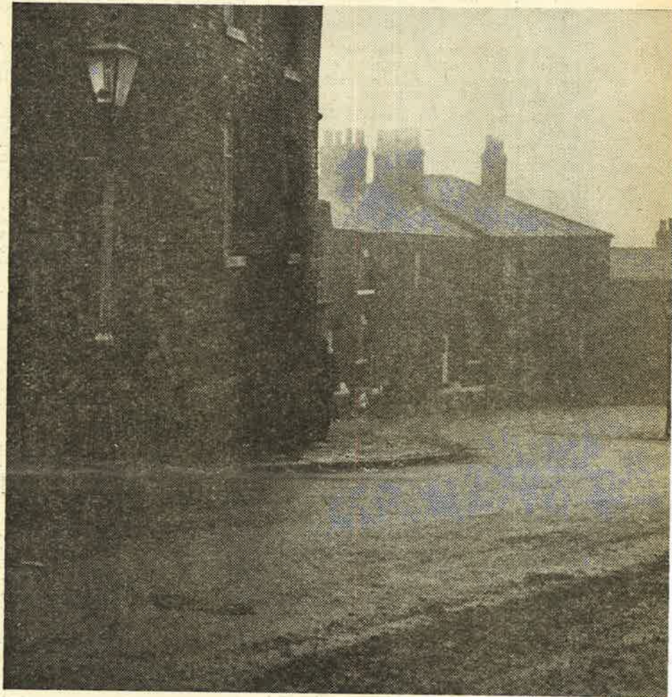
Deterioration and decay over v
