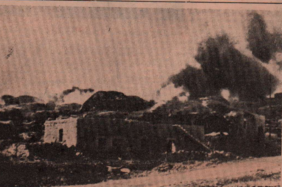
Arab homes being blown up this week on the west bank of the Jordan by the Israelis as an indiscriminate retaliation for the death of an army officer.
