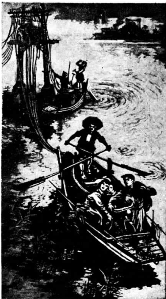
Power Line for Rural Communes
