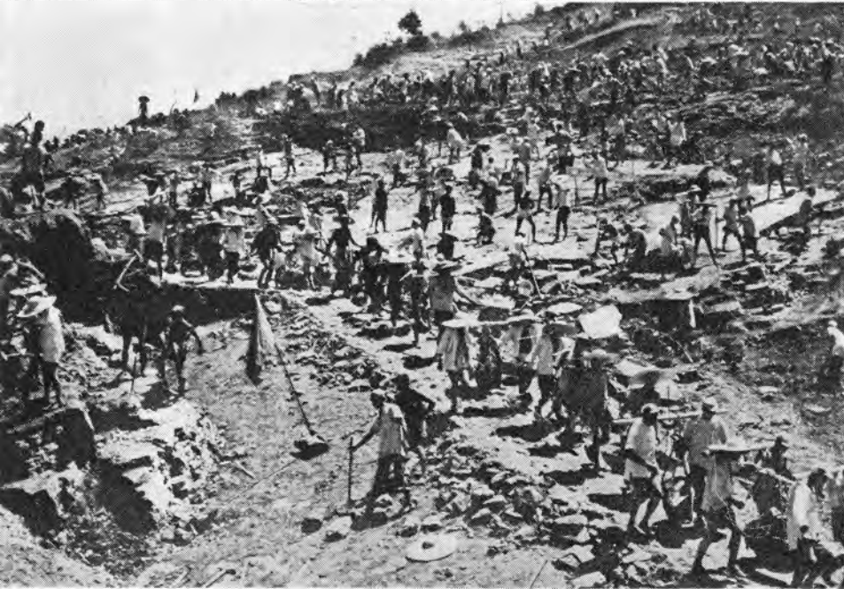
Thousands of peasant builders bring ballast for the new line
