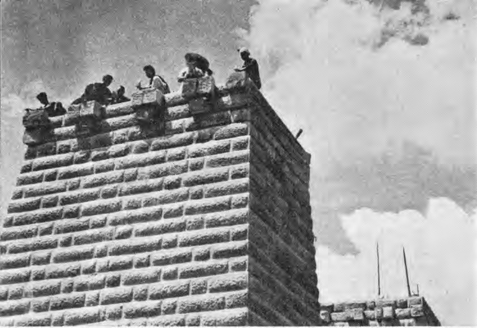
Raising pylons for the Shouchi river bridge
