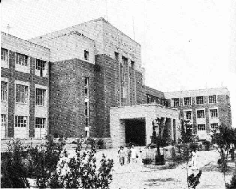
The Hospital's main facade
